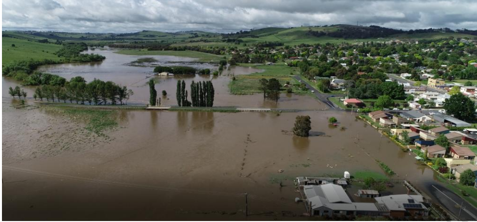
Plate B1.5 – Looking south along the western (right) overbank of the Belubula River from its confluence with Abattoir Creek (Taken on 14 November 2022 at 19:27 hours).
