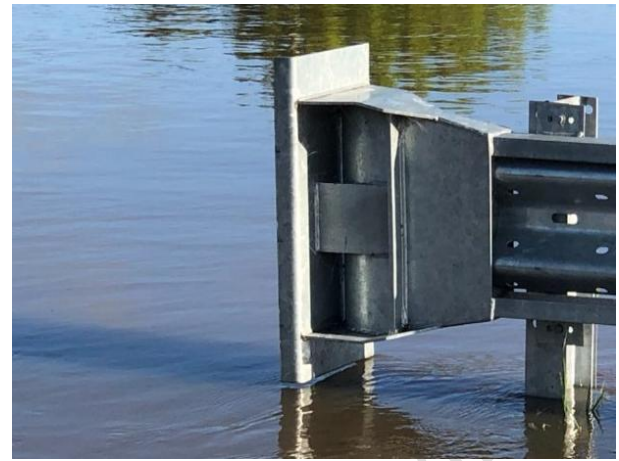
Plate B1.2 – Zoom in of Plate B1.1 showing flood level at the Glasson Bridges. The flood was observed to peak approximately 3 inches (76.2 mm) higher than the flood level in the photograph, three hours prior to it being taken.
